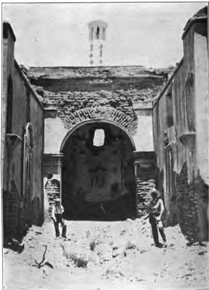
CONSTRUCTION OF ARCHES, SAN JOSÉ DE TUMACACORI, looking towards the Apse.
